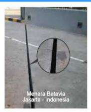
$KM\ BITU-STRIP\ as\ Connection/\ Separator\ in\ the\ building\ expansion\ joints,\ catering\ for\ shear\ \&\ lateral\ movement.$
