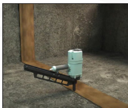
Fix the wings of the blanket to the slab every 20 cm using a pneumatic nailer.
