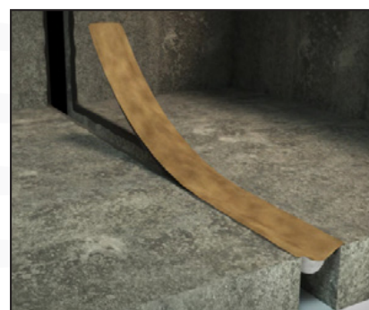
Insert the blanket into the joint.
