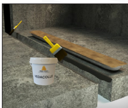
Apply the glue on both sides of the joint and on a width of 5 cm on the upper side of the concrete slab.
