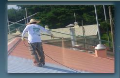
The EcoCoolRoof® System permanently adheres to virtually any type of substrate and provides protection against harmful elements throughout the life of the roof. It is fully reinforced with stitch-bonded fabric for thickness reliability, tensile strength, and flexibility. It is highly UV. resistant, chemical resistant, fire retardant, mold/ algae resistant, and vapor permeable.
